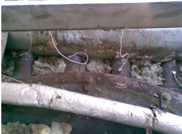
Fig. 2. Heat exchanger in a heating boiler
