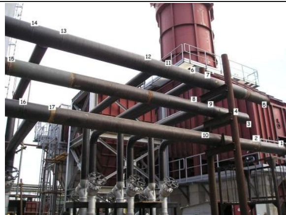
Fig. 3. Leak test points for welded pipe joints
